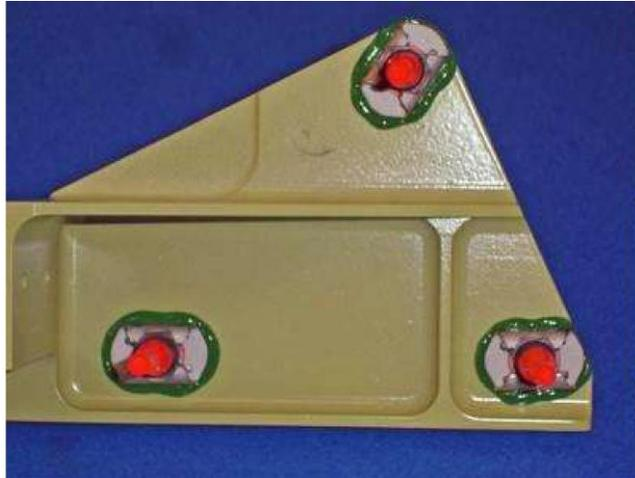
**Figure 3.** Nutplates bonded to an aluminum casting. Orange elastomer tabs passing through threaded fastener are for fixturing during adhesive cure and are removed prior to use.
